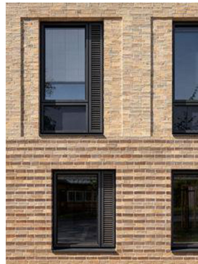
Feature brick detailing
